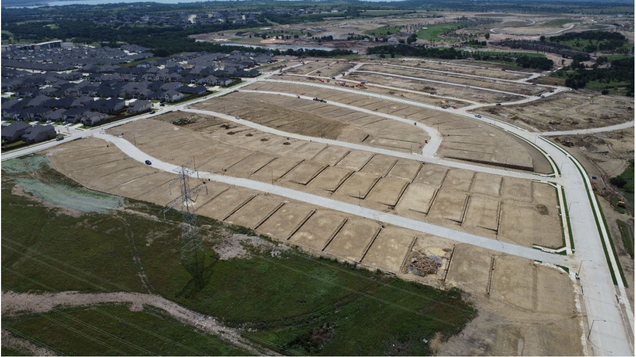
Improvement Area #5 viewed from the north
