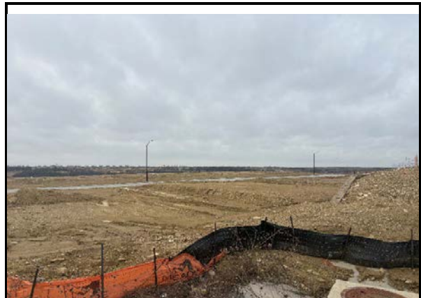
Northeast Corner of IA #5 Facing West
