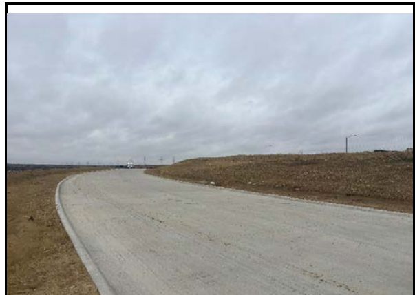
Eastern Line of IA #5 Facing North
