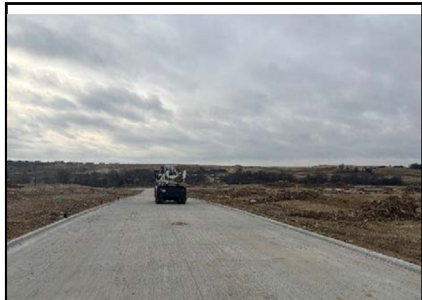
Northwest Corner of IA #4 Facing South
