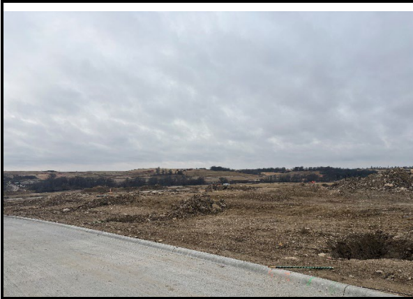
Northwest Corner of IA #4 Facing West
