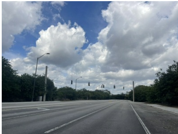
Facing north along NW 54th Ave with Block 10 on the right
