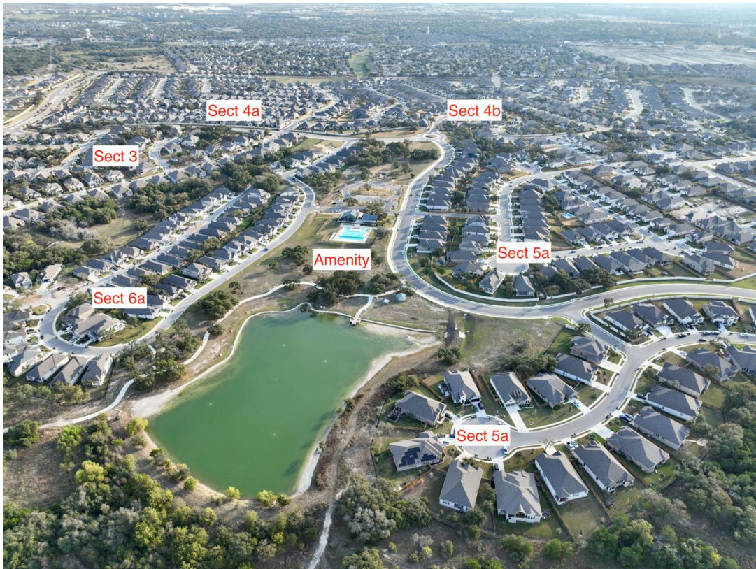
Aerial photograph of Development showing Sections 3, 4A, 4B, 5A, and 6A.
