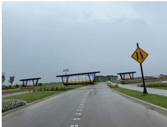
Main Entrance to Solterra Development
