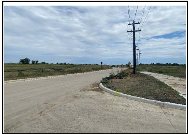
Celina Parkway Facing North
