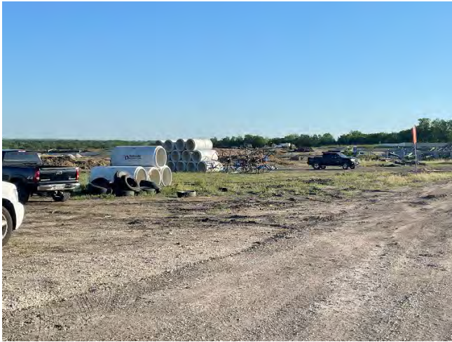
View of interior roads under construction
