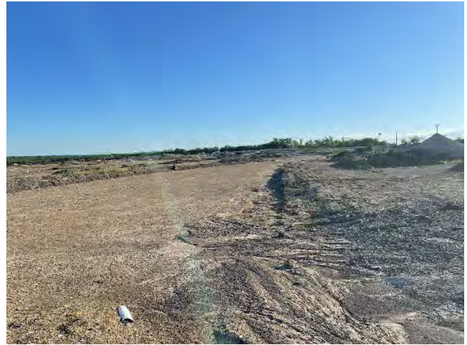
Interior view of subject showing site work
