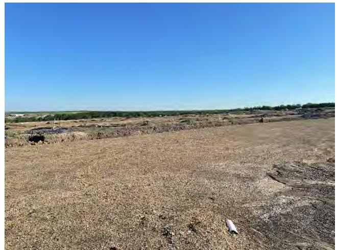
Interior view of subject showing site work
