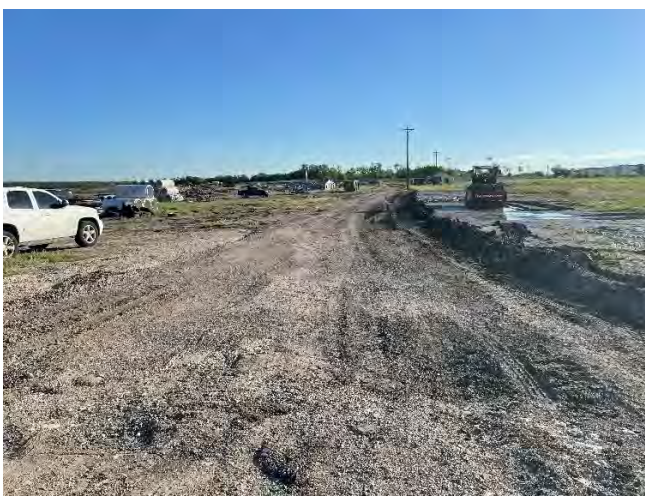
View of main entry road under construction in subject
