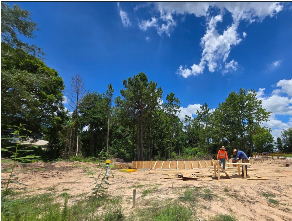
Construction Progress on East Entry Monument on Holderrieth Road
