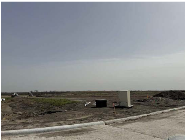
Clearview Ranch Public Improvement District, Phase 1 - North within North Zone Improvement Area #1 South side of CR-677, east of FM-1777 Royse City, Collin County, Texas
