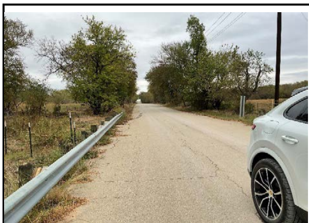
Shearer Road facing east
