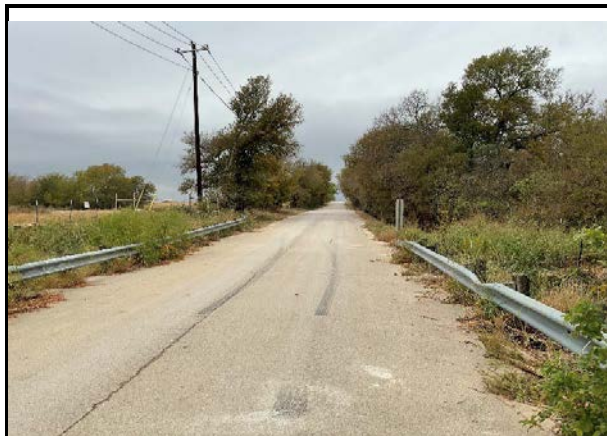
Shearer Road facing west
