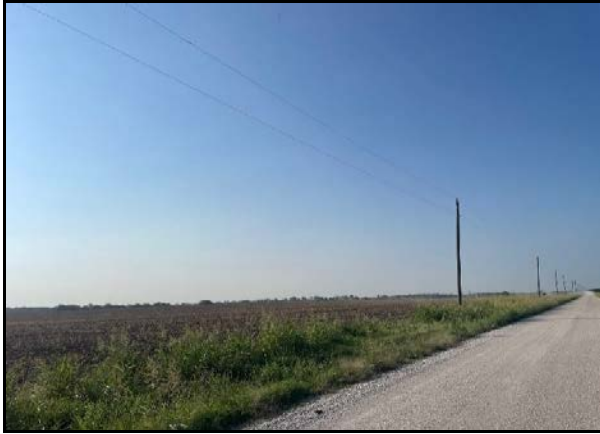
Tract 6 viewing southeast
