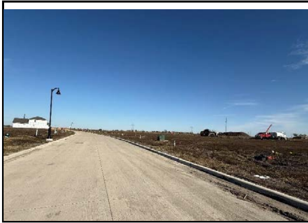
Intersection of Tule Way and Toyah Lane viewing east
