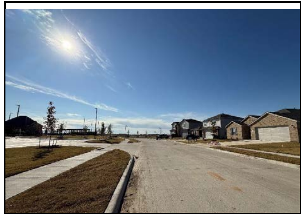
Coleta Road viewing West
