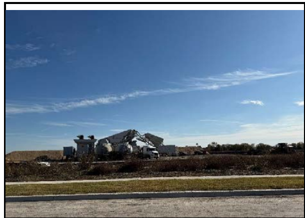
Tule Way viewing south
