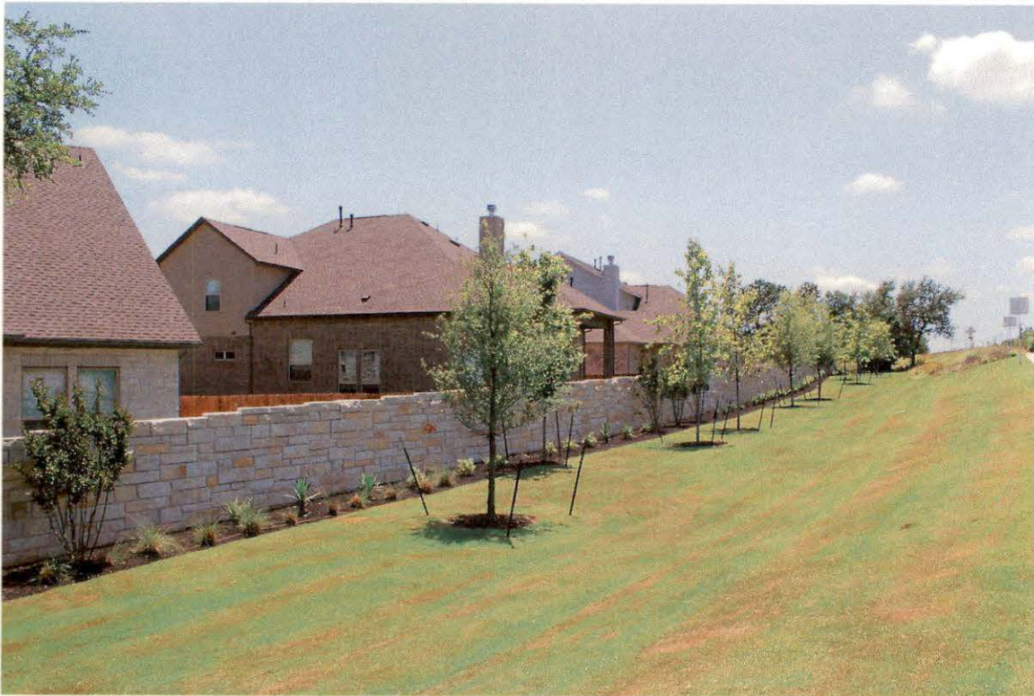
Post-Tension Rock Wall
