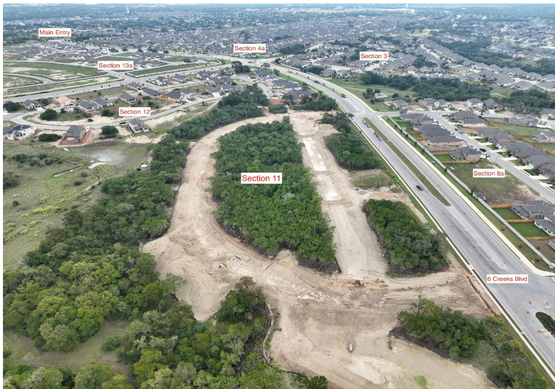
Aerial photograph of Development showing Section 11 in relation to other sections.
