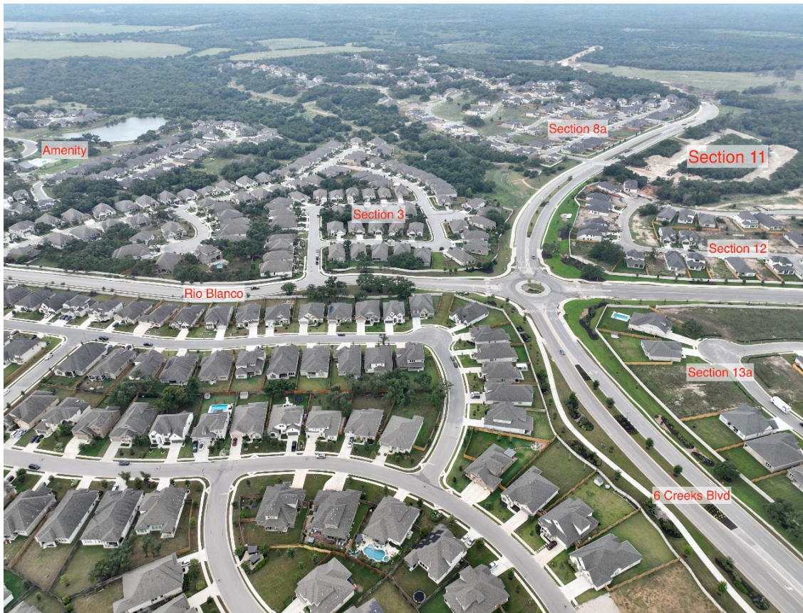
Aerial photograph of Development showing Section 11 in relation to other sections
