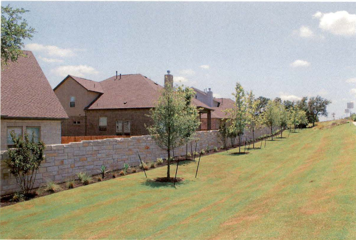
Post-Tension Rock Wall
