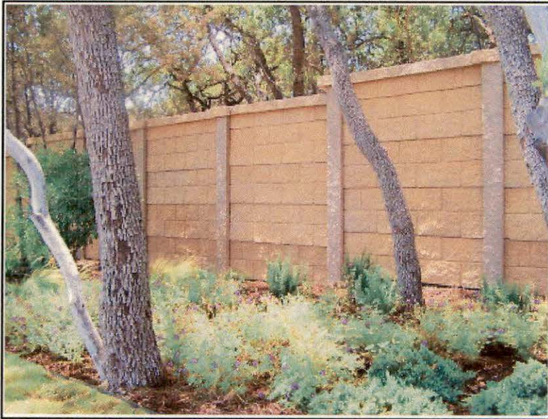
Split-Face CMU Style Concrete Fence
