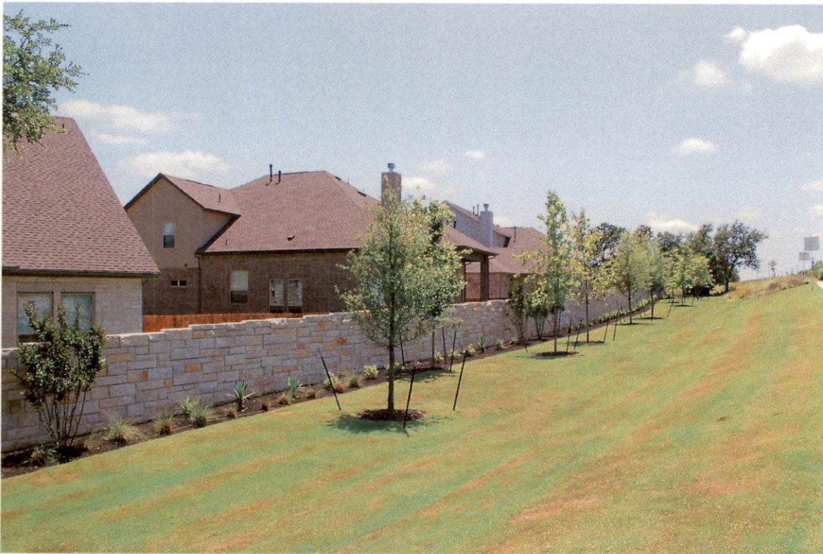
Post-Tension Rock Wall
