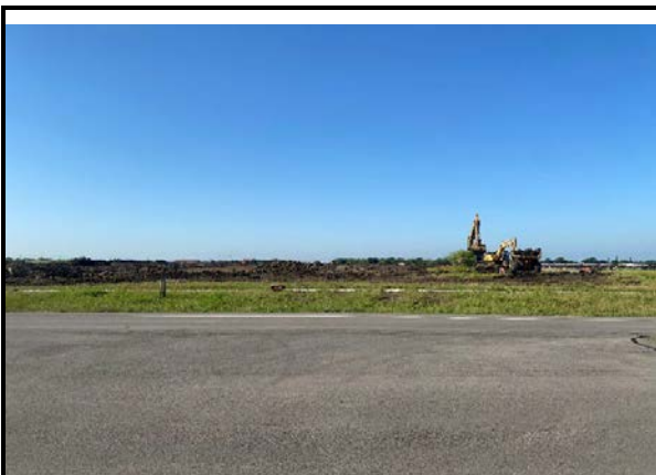
Northwest corner of subject facing south
