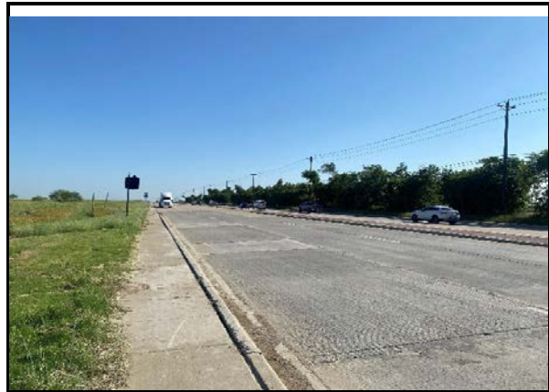
Facing north on West FM Road 720
