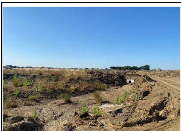
North border of subject facing south
