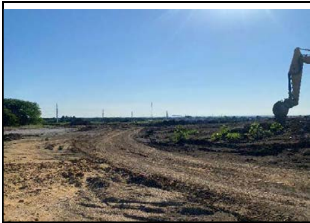
Northwest corner of subject facing east
