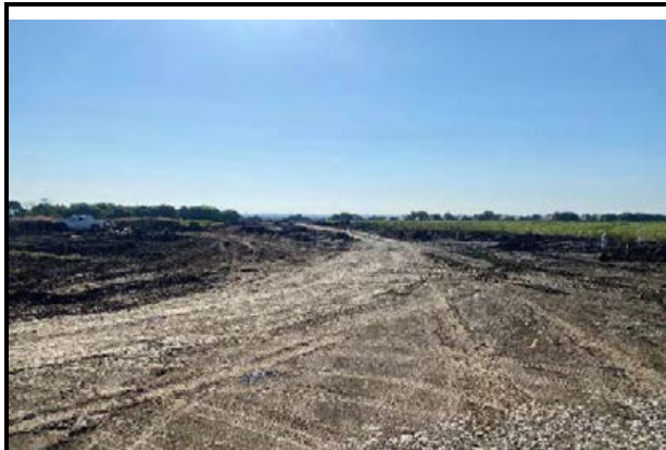
Southwest corner of subject facing east
