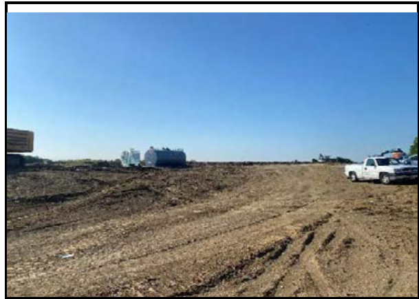
Northwest corner of subject facing south
