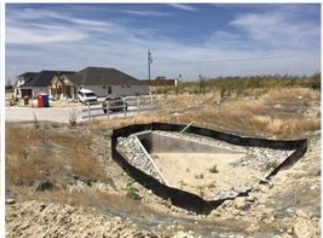
Drainage Culvert with Headwalls and Rip Rap Rock near Boundary of Improvement Areas #2 and #3
