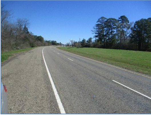
S.H. 30 facing east
