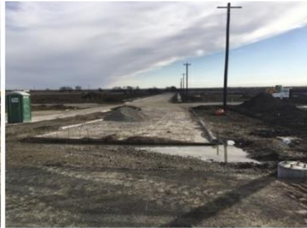
Main Entrance Off FM 1385 At Phase 1
