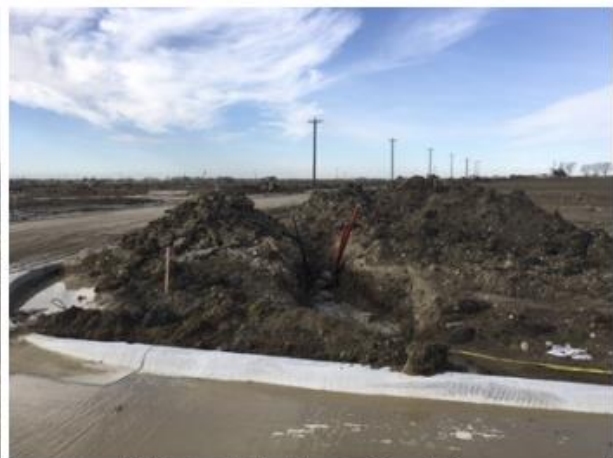
Utility Installation Nearing Completion
