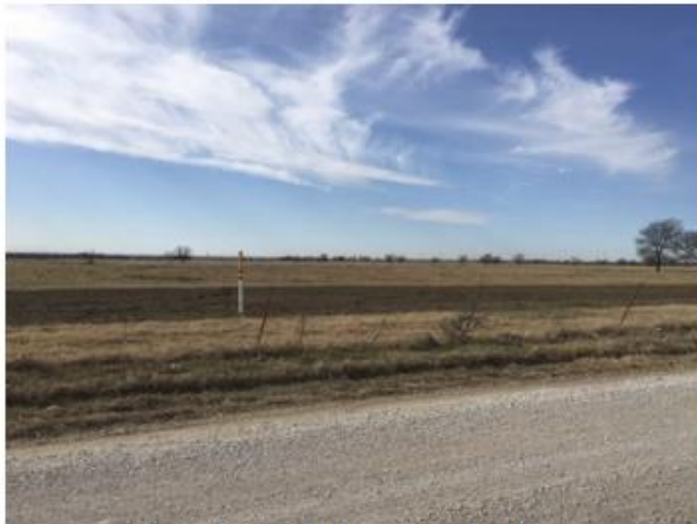
Phase 2 Showing Natural Gas Pipeline
