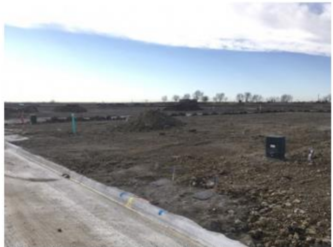
Water, Sanitary Sewer, Electric, Natural Gas, Telecom And Storm Sewer Appear To Be Complete
