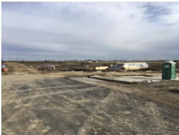
View North At Main Entrance Looking Across Phase 1
