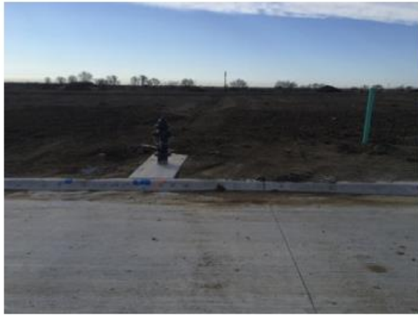
Fire Hydrants Installed
