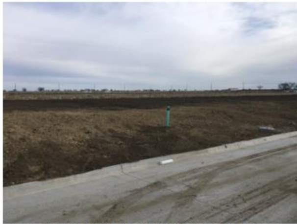
Stone Retaining Walls Are On Multiple Streets In Phase 1
