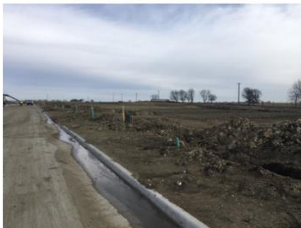
Utility Trenching In Phase 1
