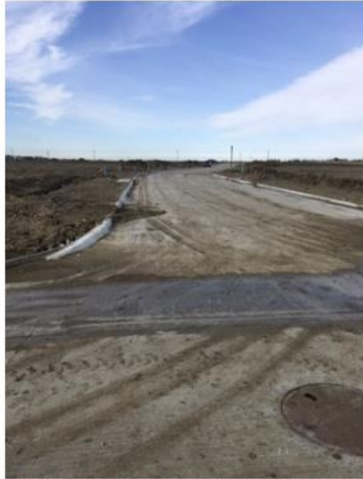
Roads Are Concrete Paved With Concrete Curbs And Storm Sewer
