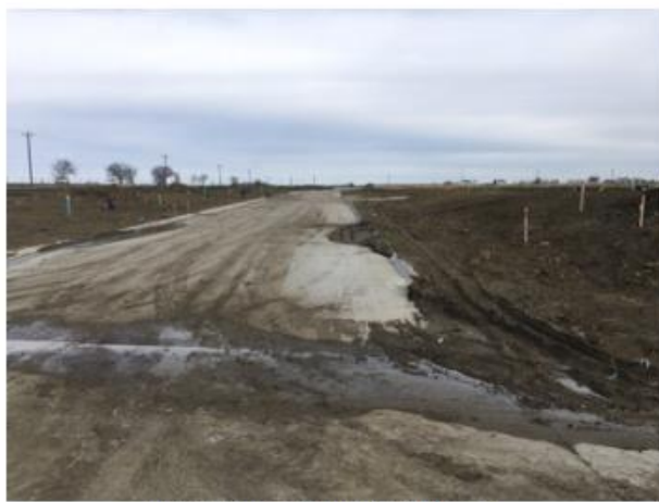
Paved Concrete Roads In Phase 1
