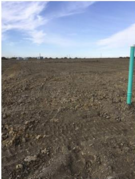
Graded Lots In Phase 1
