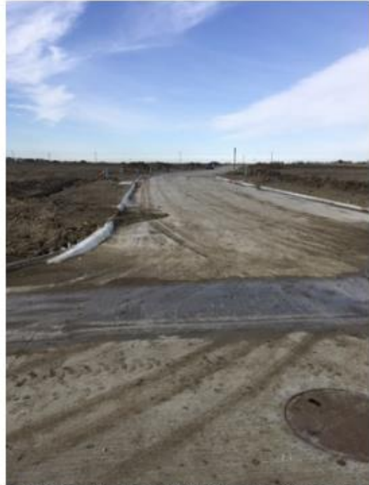
Roads Are Concrete Paved With Concrete Curbs And Storm Sewer
