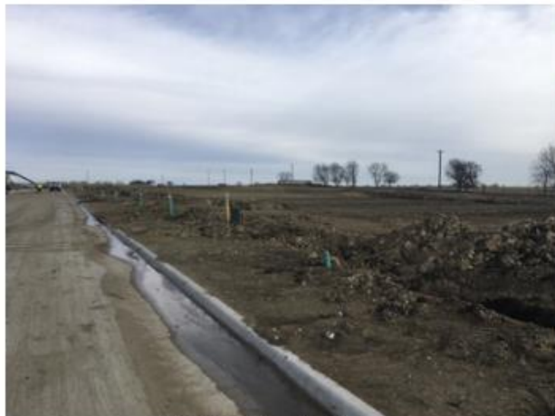
Utility Trenching In Phase 1
