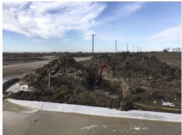
Utility Installation Nearing Completion
