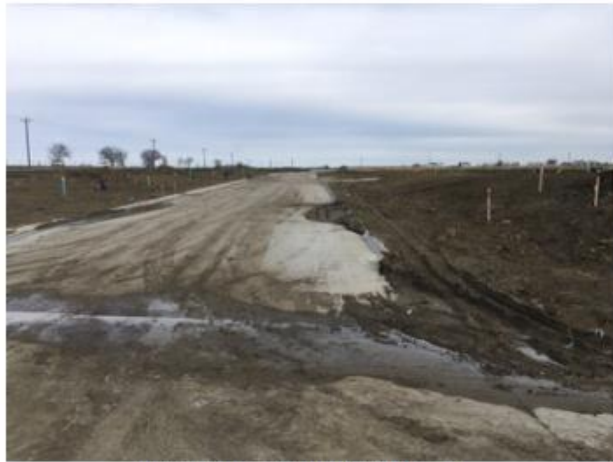
Paved Concrete Roads In Phase 1
