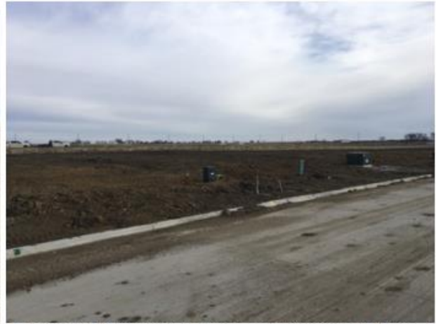
Retaining Walls Installed, Utilities Almost Complete In Phase 1
