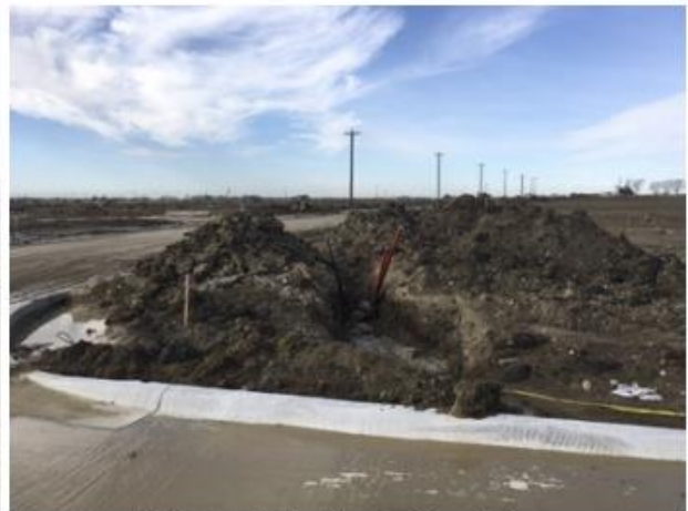
Utility Installation Nearing Completion
