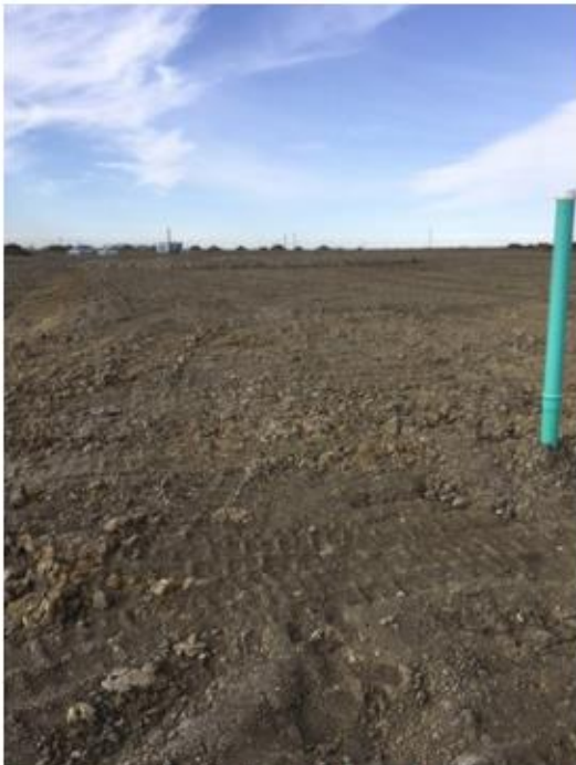
Graded Lots In Phase 1
