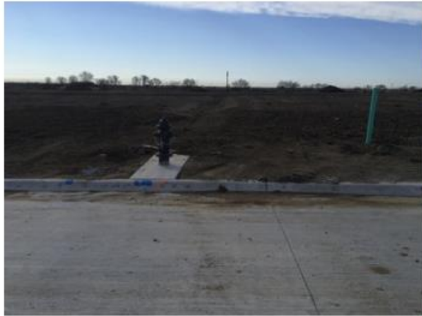
Fire Hydrants Installed
