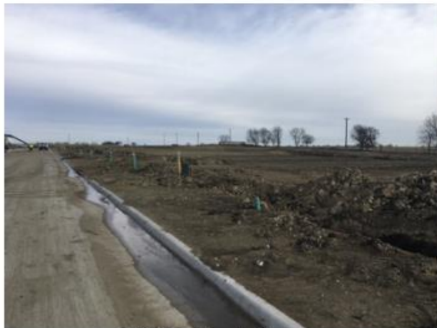
Utility Trenching In Phase 1
