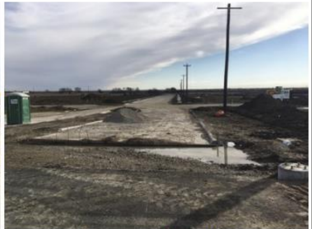
Main Entrance Off FM 1385 At Phase 1
