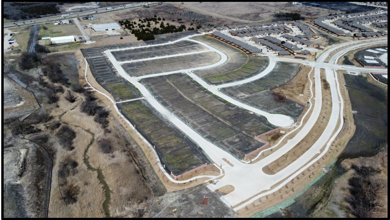
Developed Lots in Phase 3A2 (Facing Northeast)
