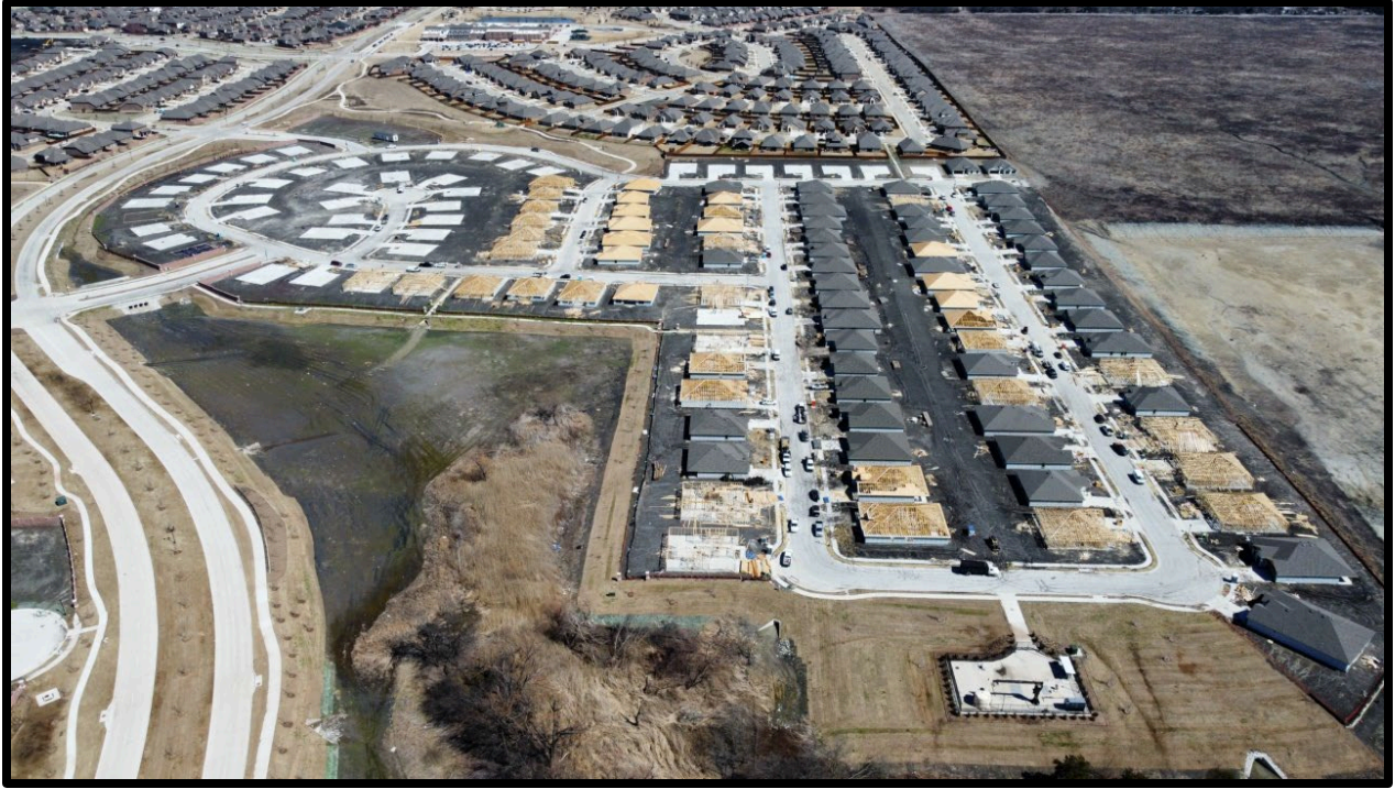
Homes under Construction in Phase 2A
