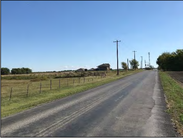
Looking Northeast across Pod 2B from Watkins Rd. (CR541)
