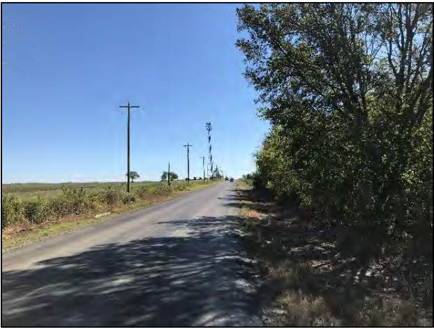
Looking East down Watkins Rd. (CR541) 2B & 2D on the Left (Cell Tower as reference point)
