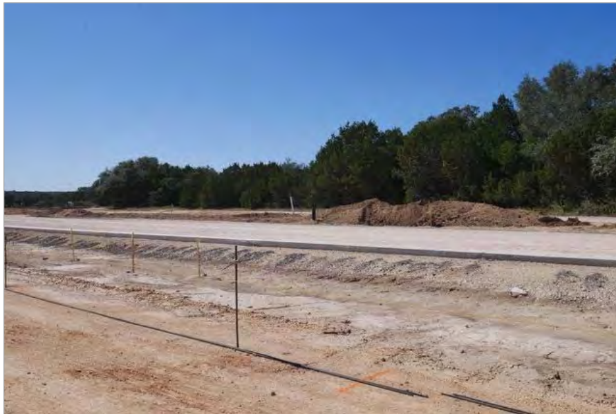
Trunk Road Under Construction
