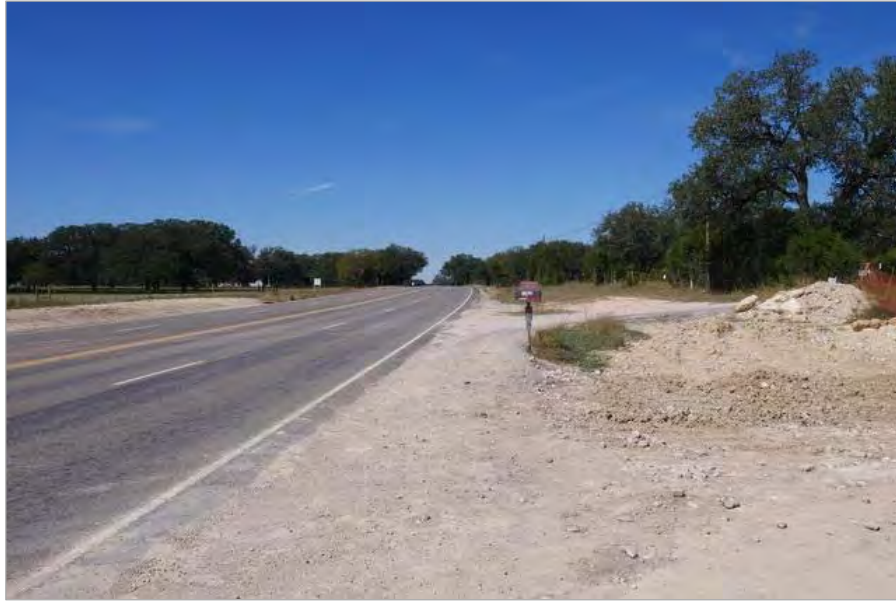
State Highway 29 Looking West – Subject at Right
