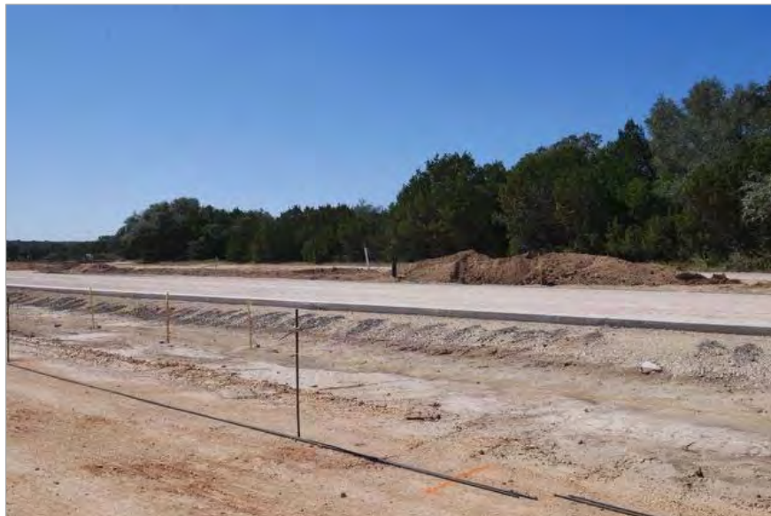
Trunk Road Under Construction
