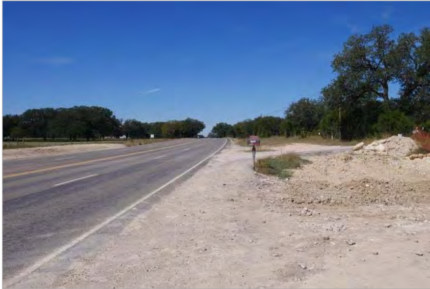
State Highway 29 Looking West – Subject at Right
