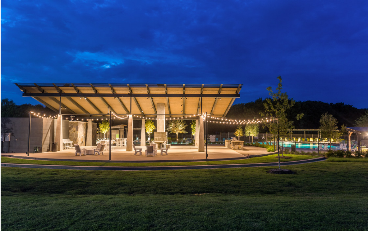
Exterior of Pool-Pavilion
