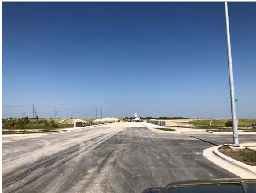
Infrastructure with Bridge Over Floodplain
