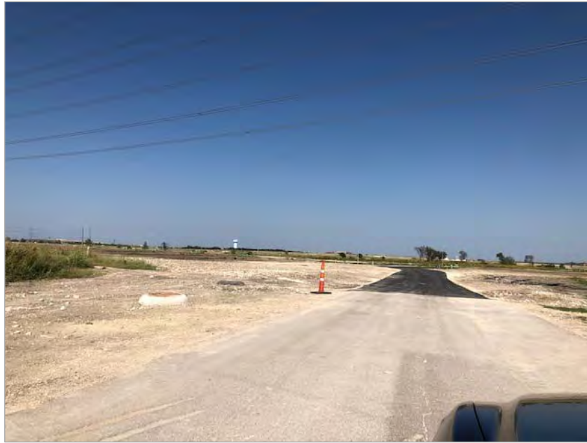
Secondary Entrance Off Ed Schmidt Boulevard
