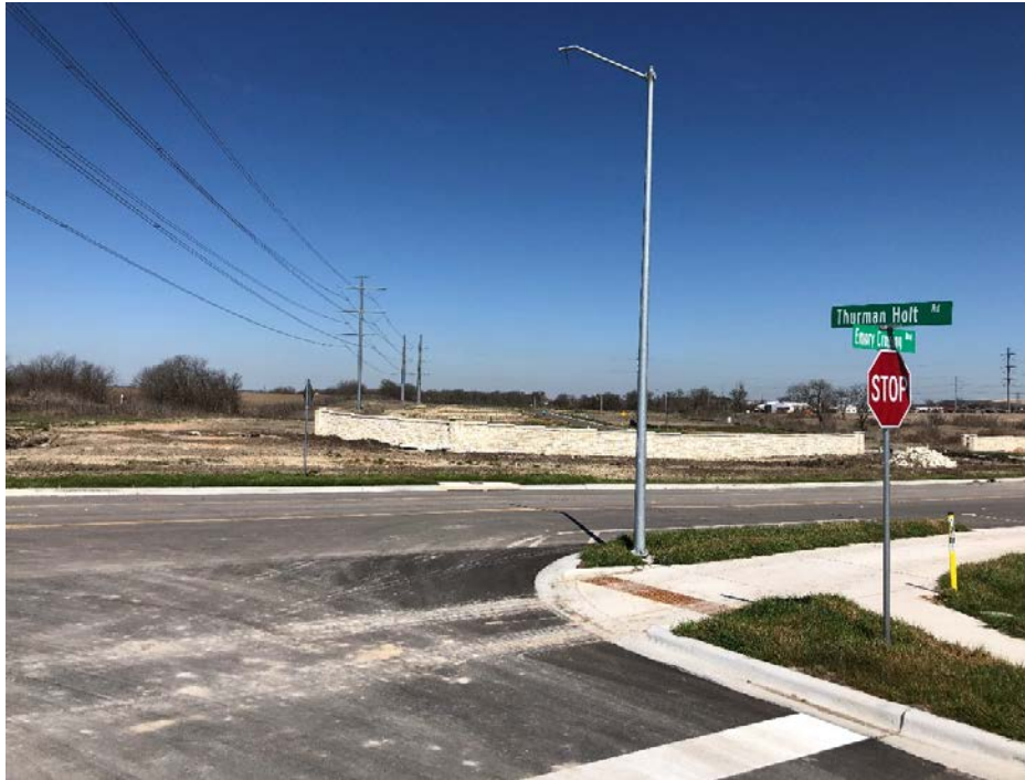
Intersection of Emory Crossing Blvd and Thurman Holt Rd
